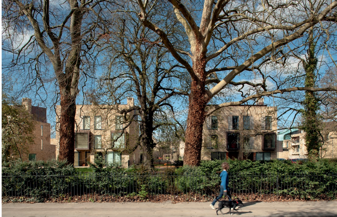
Osiedle Accordia, widok od ulicy, proj. Feilden Clegg Bradley Studios, Maccreeanor Lavington Architects, Alison Brooks Architects.
